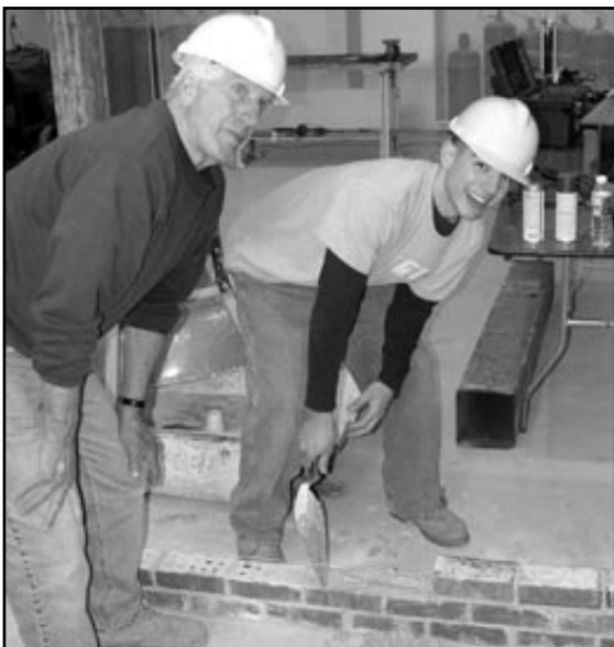
Construction Career Day Steve Bevilaqua learns to apply mortar
